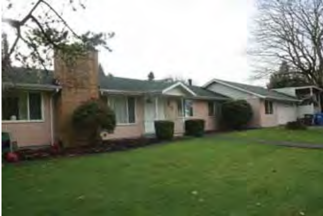
View to the southwest North (front) elevation 2015
