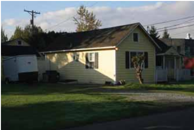
View to the southeast North (front) and east elevations 2015
