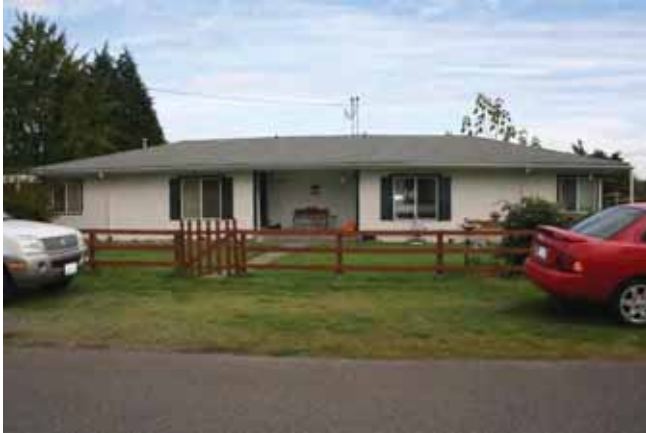
View to the east West (front) elevation 2015
