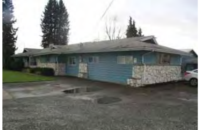
View to the southeast North (front) and west elevations 2015
