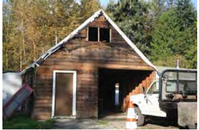
View to the south Garage, north elevation 2015
