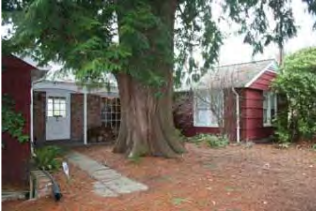
View to the southeast Erickson House, east and south elevations 2016
