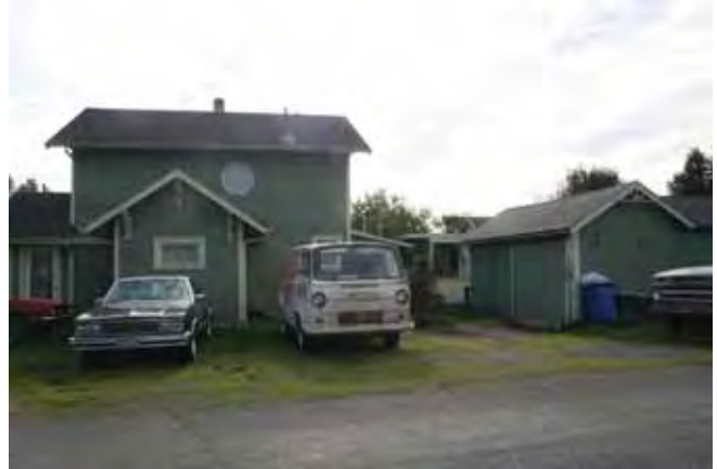
View to the south North elevation and sheds 2015
