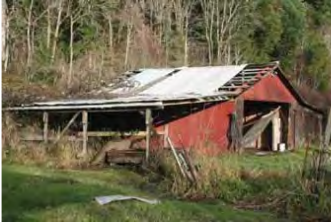
View to the northeast Shed, west and south elevations 2015
