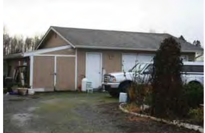
View to the southwest Garage, north and east elevations 2015
