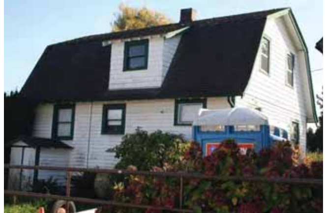
View to southeast House, north and west elevation 2015
