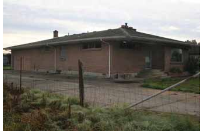
View to the southeast West (front) and north elevations 2015
