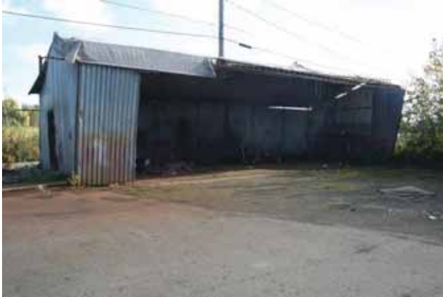
View to the east Shed 1, west elevation 2015
