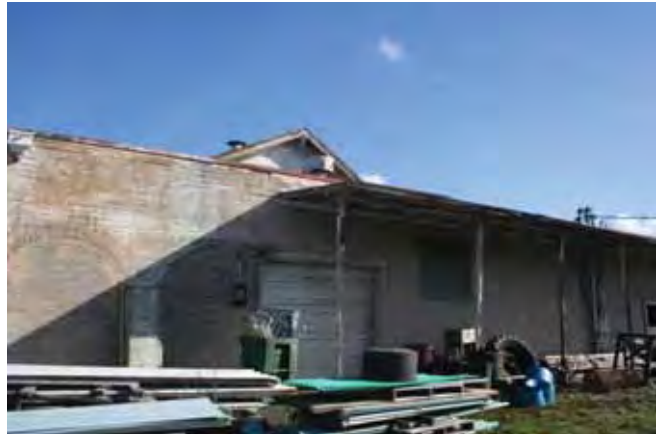
View to the southeast Brick building, west elevation 2015
