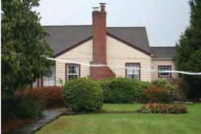
View to the east West (front) elevation 2016
