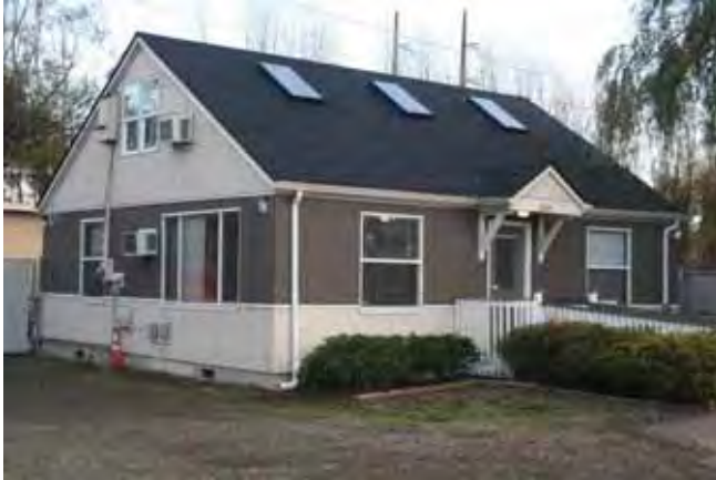
View to the northeast South (front) and west elevations 2015
