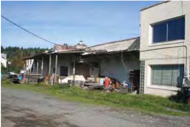
View to the northeast Brick building, offices, west elevation 2015
