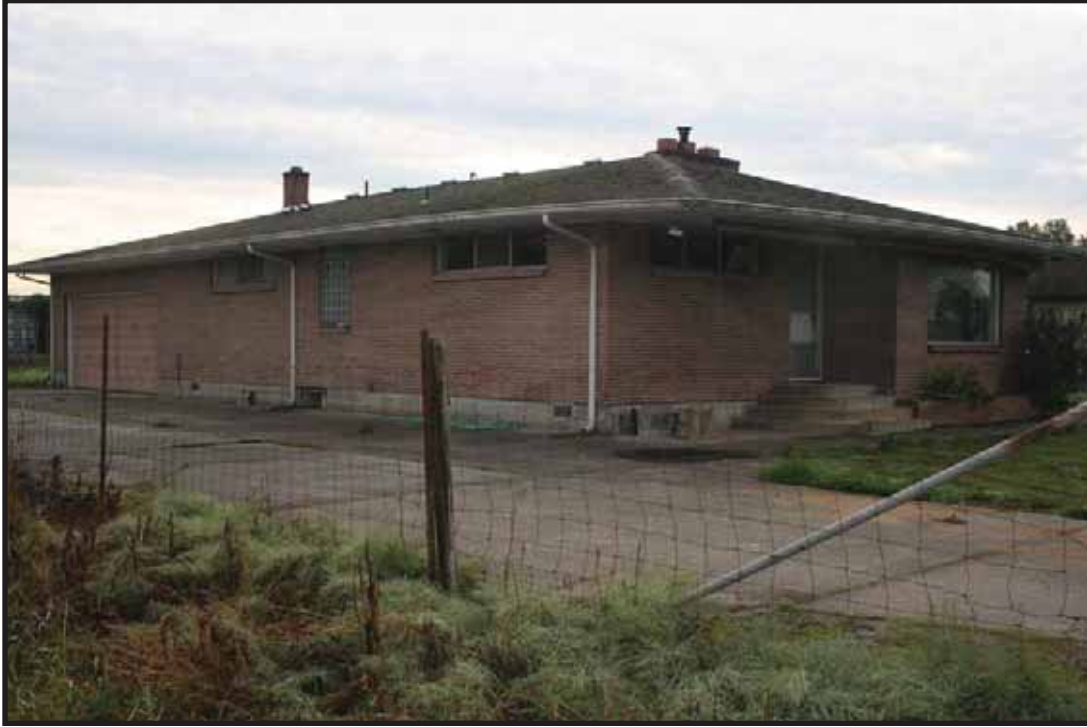
Figure 13. Boitano residence, 4403 Freeman Road E, west (front) and south elevations, view to the northeast.
