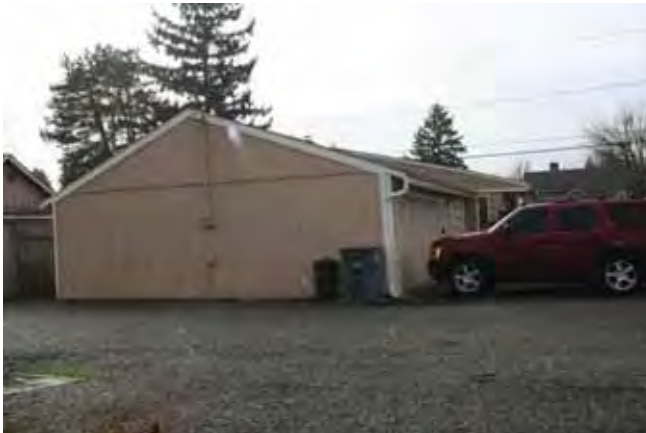
View to the southwest North (front) and east elevations 2016
