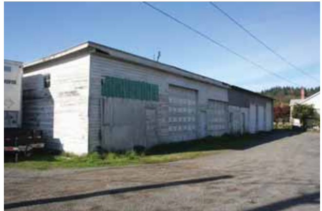
View to the northwest Wood frame vehicle garage, east elevation 2015
