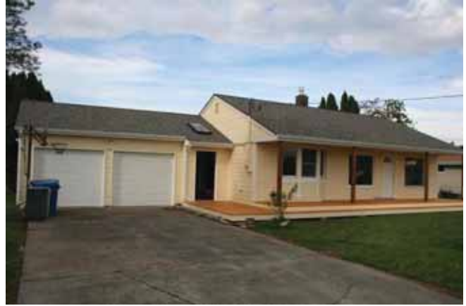
View to the northwest East (front) and south elevations 2015
