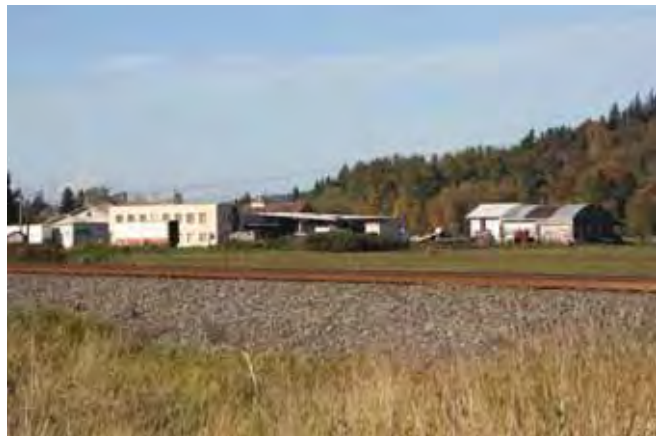
View to the northwest Overview 2015
