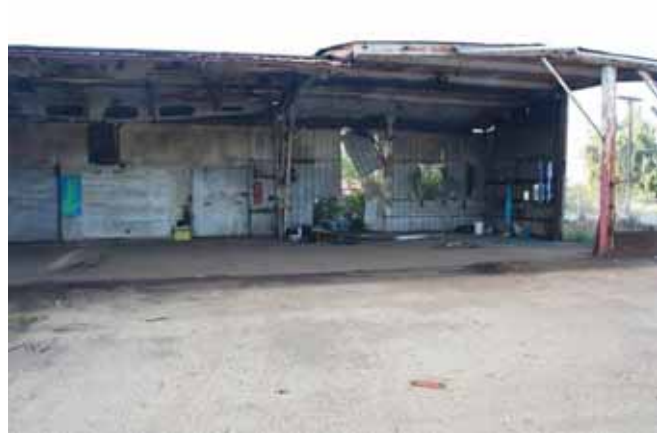
View to the west Shed 2, east elevation 2015
