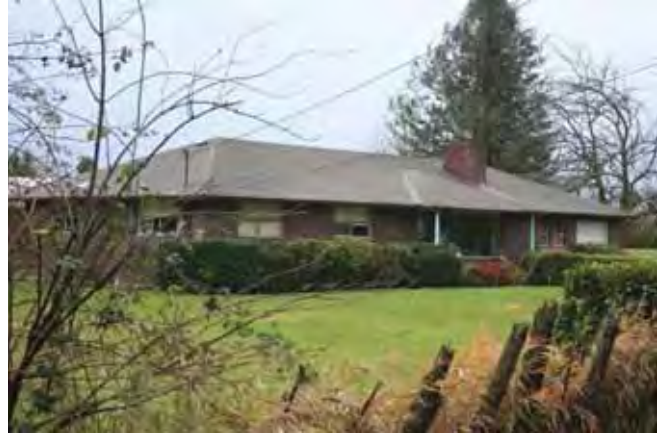
View to the southwest North (front) and east elevations 2015
