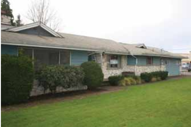
View to the southwest North (front) elevation 2015
