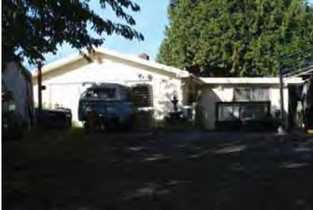
View to the north South (front) elevation 2015
