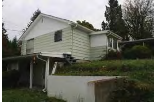
View to the northeast West and south (rear) elevation 2015
