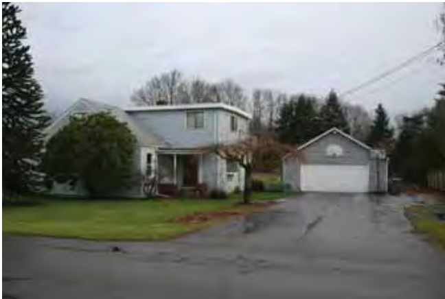
View to the northeast House, west and south elevations, garage, west elevation 2015
