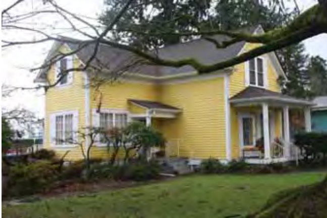
View to the southeast West (front) and north elevations 2016
