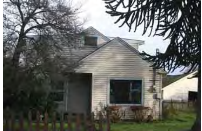
View to the east West (front) elevation 2015
