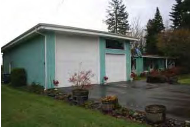
View to the southeast Garage, west elevation 2016
