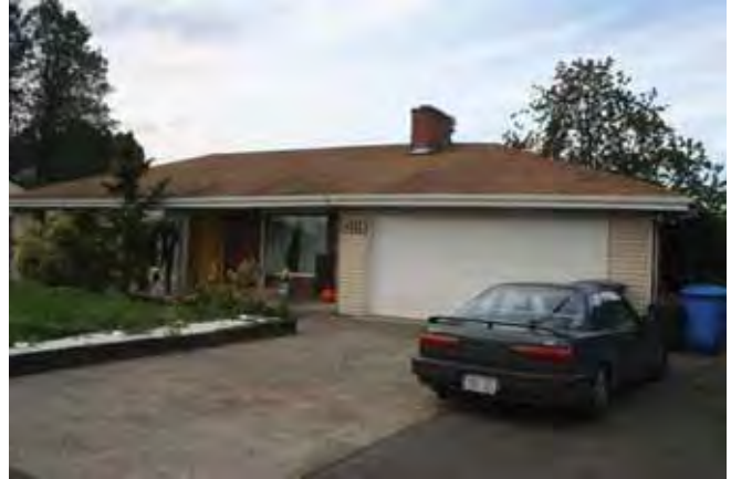
View to the southwest East (front) elevation 2015
