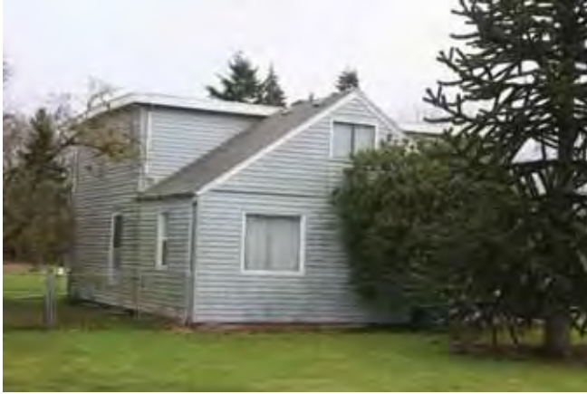
View to the southeast west and north elevations 2015
