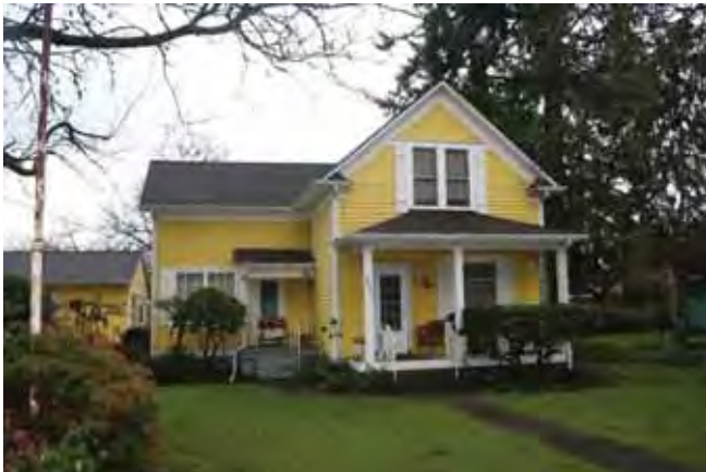
View to the east West (front) elevation 2016
