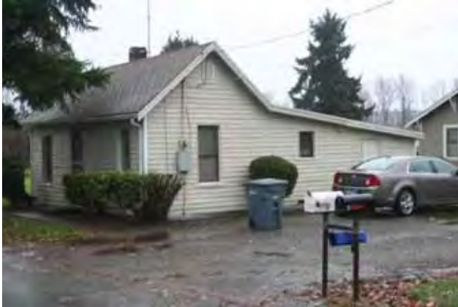
View to the northeast West (front) and south elevations 2016
