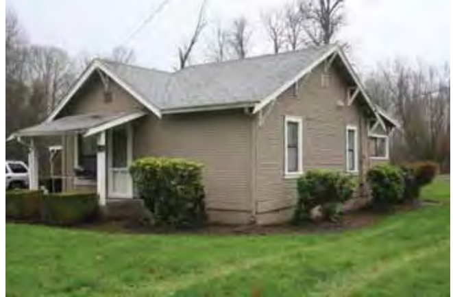
View to the southeast North (front) and west elevations 2016
