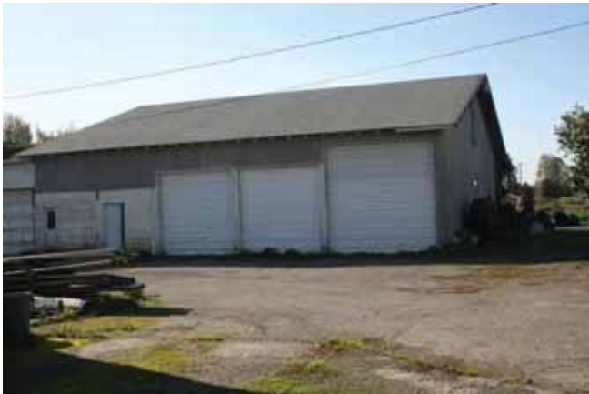
View to the northeast Metal vehicle garage, west elevation 2015
