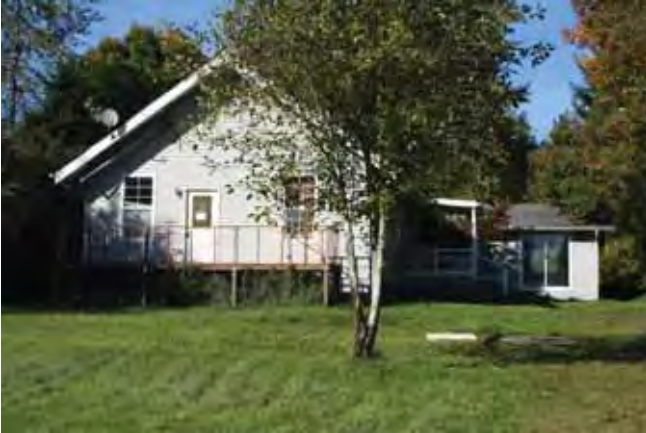
View to the north South (front) elevation 2015
