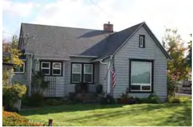
View to the southeast West (front) and north elevations 2015
