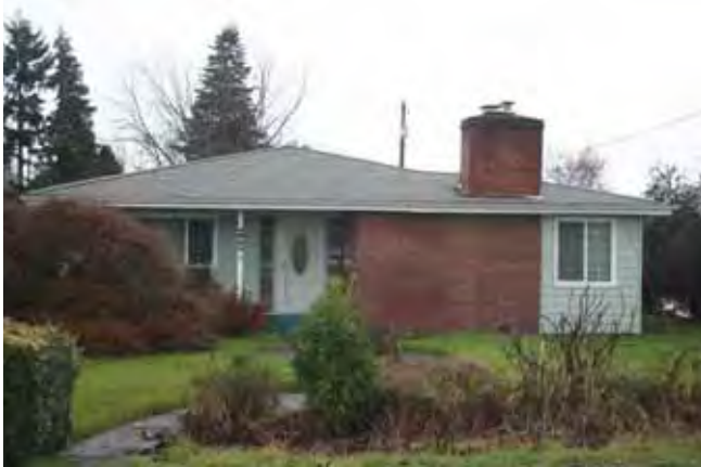
View to the east West (front) elevation 2015
