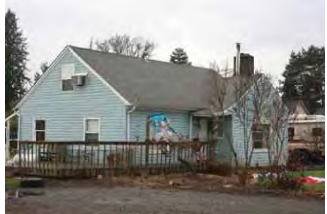
View to the southwest North (front) and east elevations 2015
