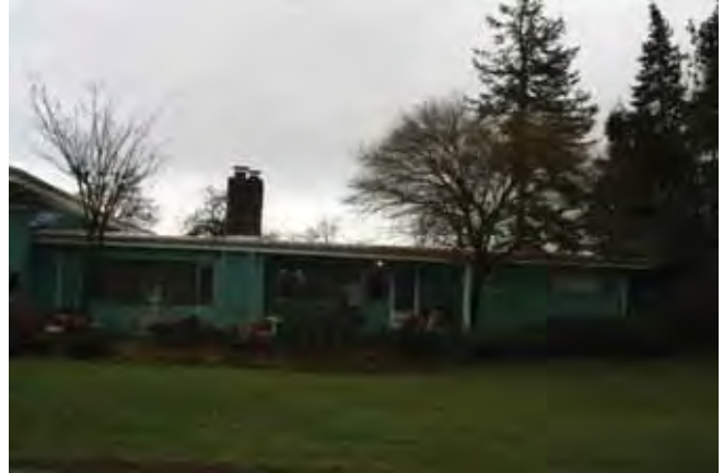
View to the east West (front) elevation 2016
