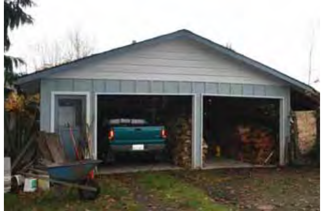
View to the west Garage, east elevation 2015
