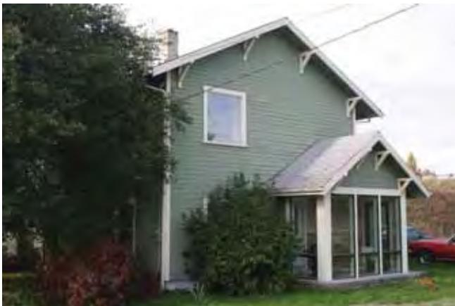
View to the northwest East (front) elevation 2015
