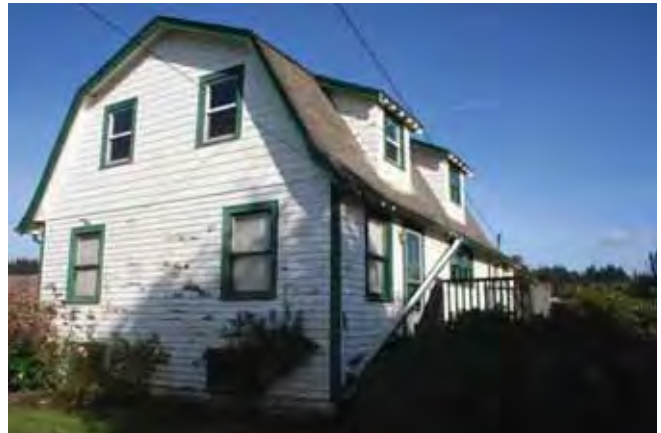
View to the northeast House, south (front) and west elevations 2015
