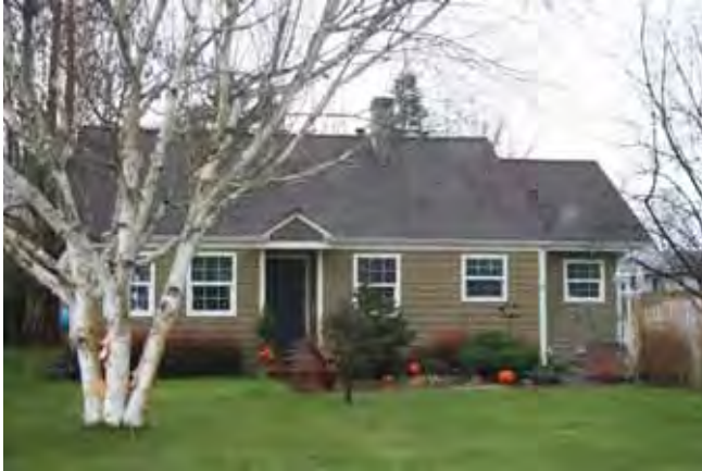
View to the east West (front) elevation 2015
