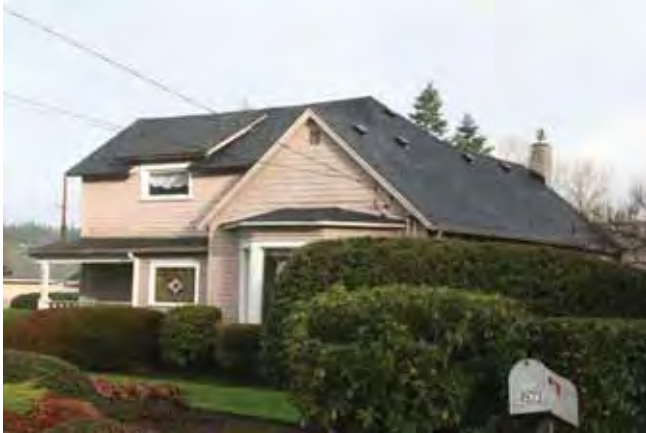
View to the northeast Front (west) elevation 2015
