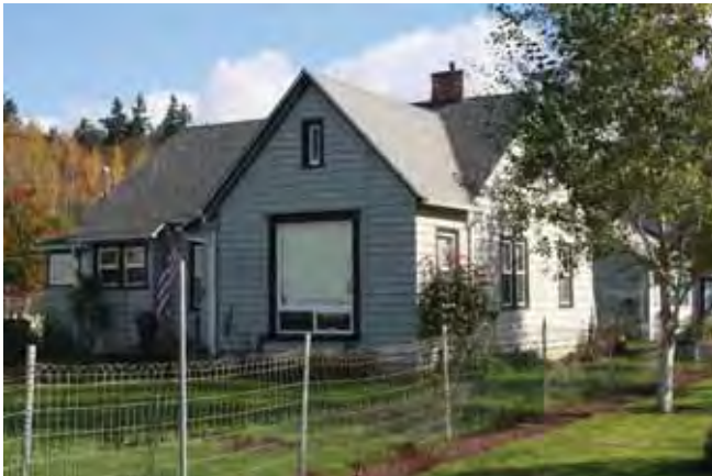
View to the northeast West (front) and south elevations 2015
