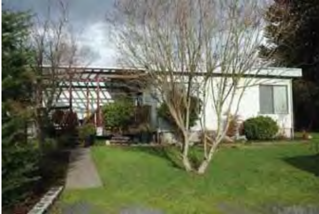
View to the north South (front) elevation 2015
