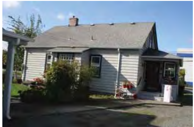
View to the southwest East (rear) and north elevations 2015
