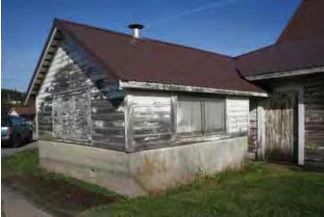
View to the northeast Milk shed, west and south elevations 2015
