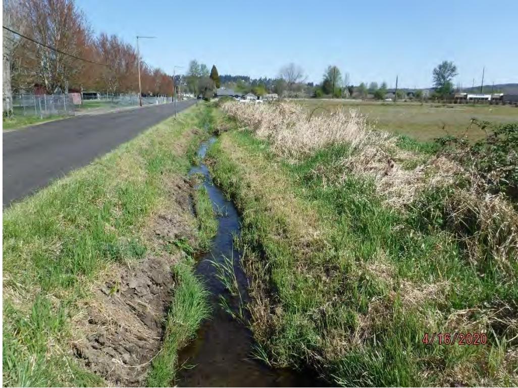
View northerly along Deer Creek near the southwestern corner of the project site.
