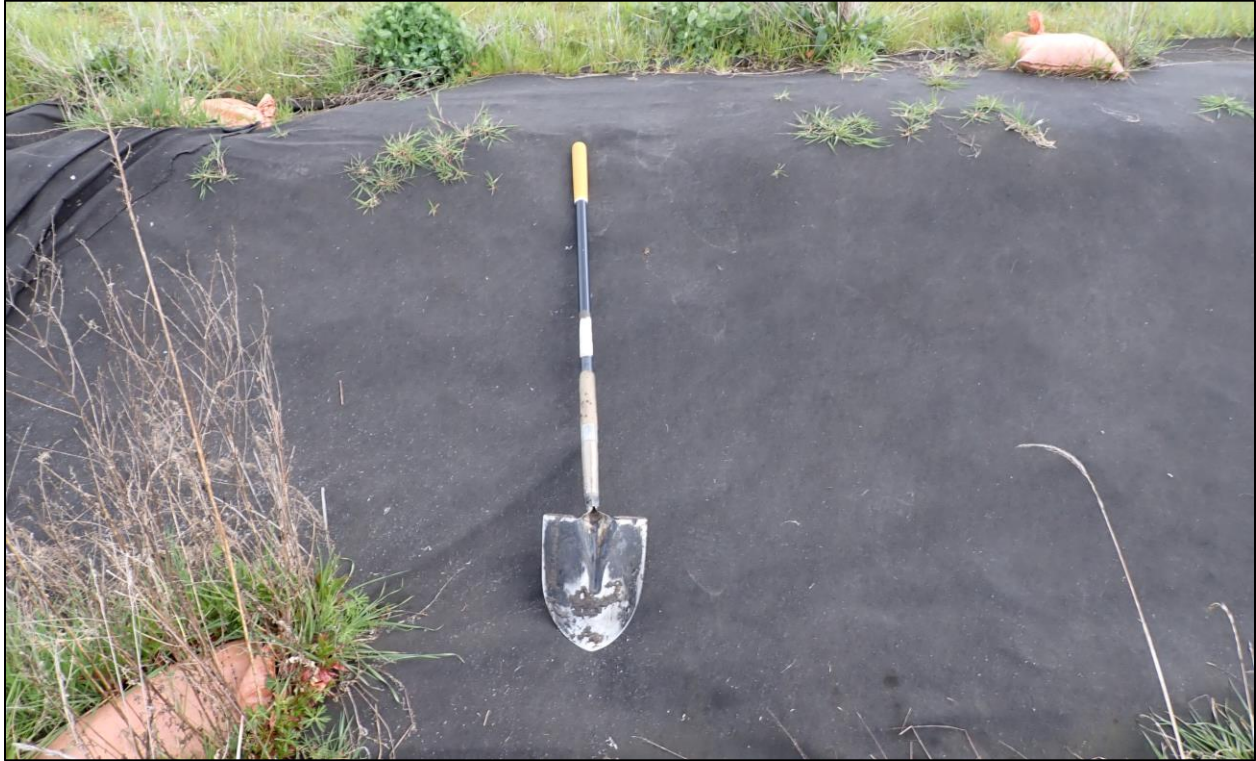
Photo 4. Landscaping fabric containing the fill along the eastern project boundary.
