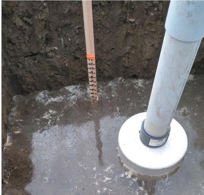
Figure 10: Infiltration Test in Progress PIT 6, Lot E
