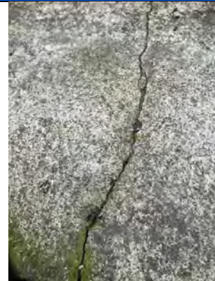
Hairline Crack in Concrete
