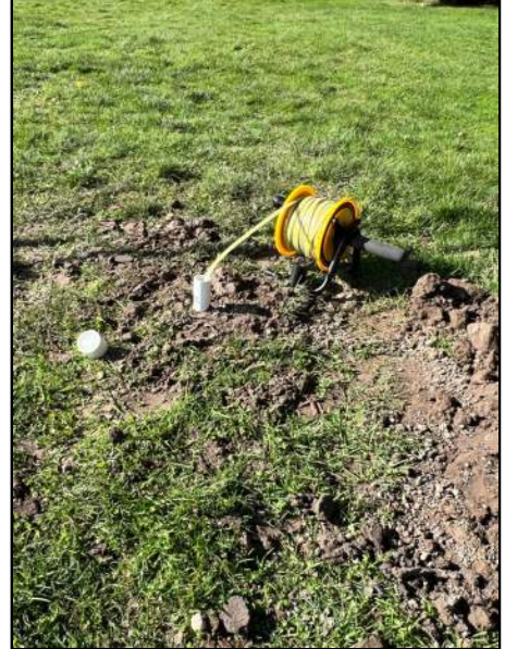
Backfill and Install Groundwater Monitoring
