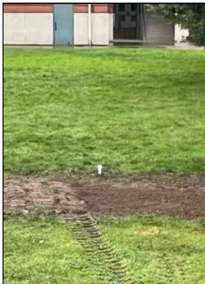
Backfill and Install Groundwater Monitoring
