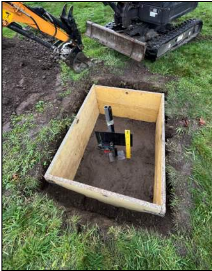
3-feet x 4-feet x 2-feet PIT
