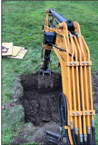
Overexcavate to Verify Groundwater Mounding
