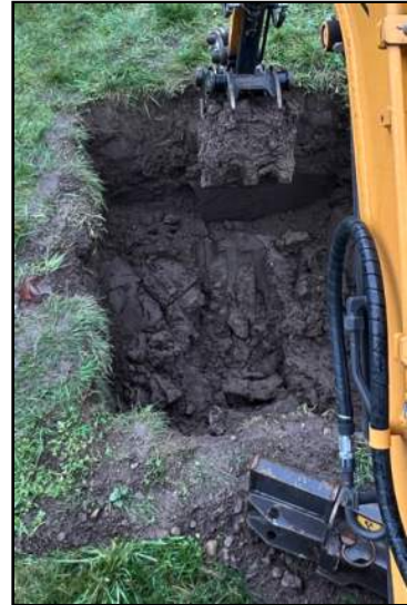
Overexcavate to Verify Groundwater Mounding
