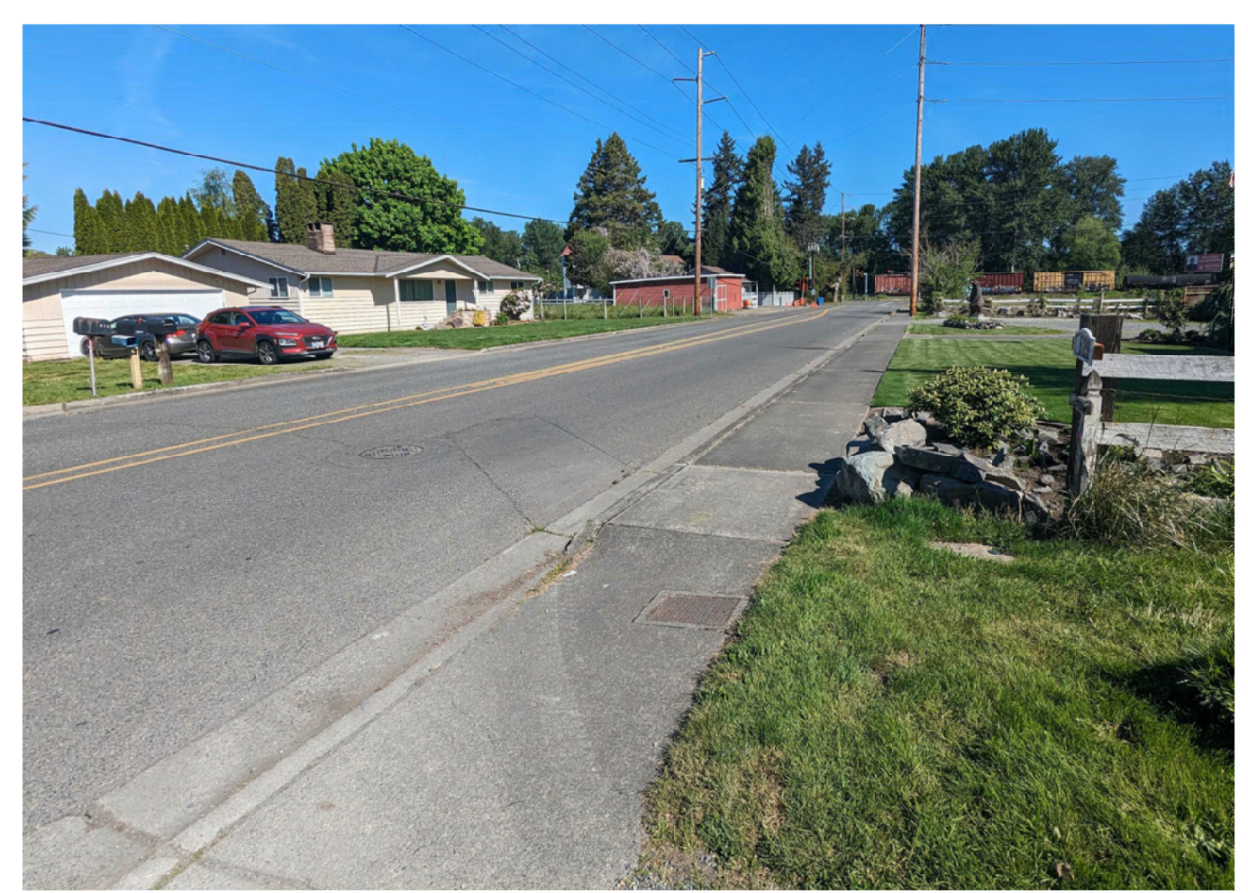
LOOKING NORTH FROM DRIVEWAY
