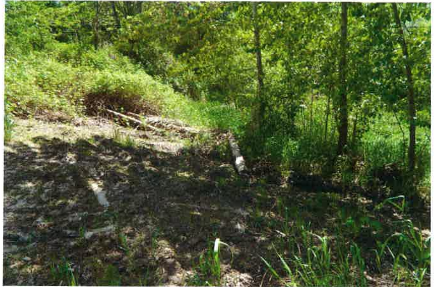
Northeast wall of retention pond
