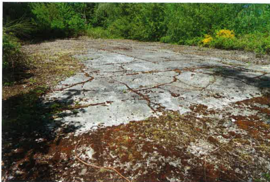
Foundation of Storage Barn
