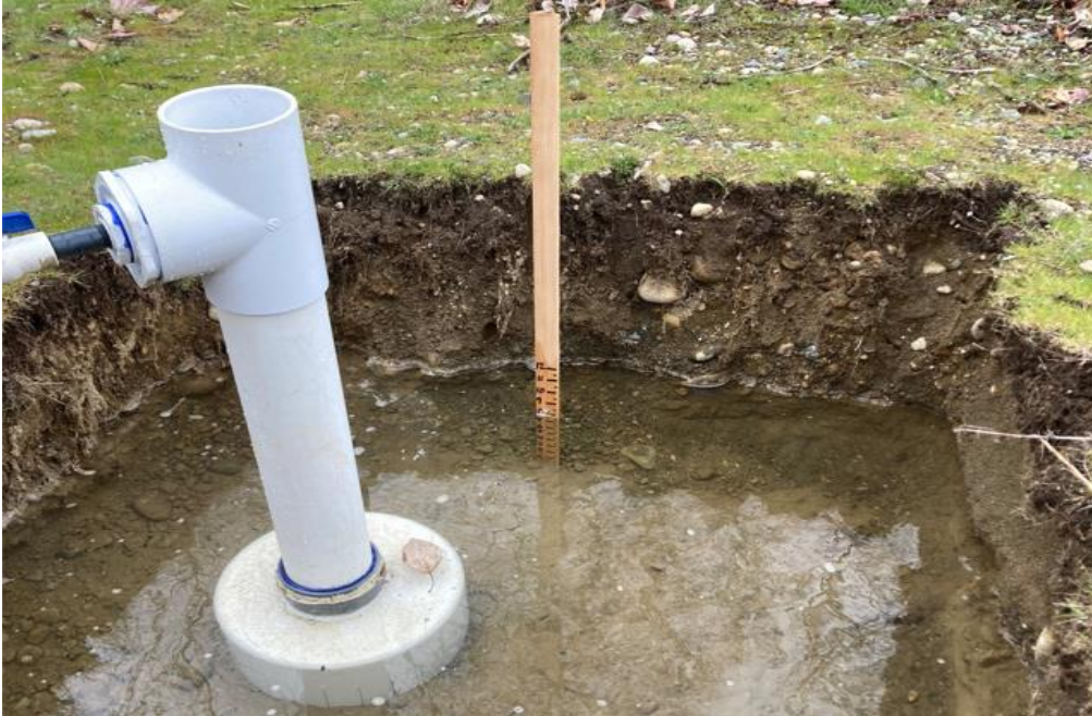
Figure 6: Infiltration Test in Progress PIT 1, Lot C
