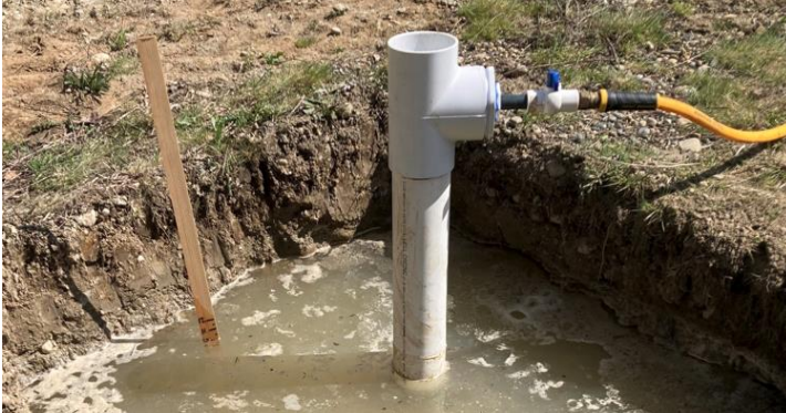
Figure 7: Infiltration Test in Progress PIT TEST 2, Lot C
