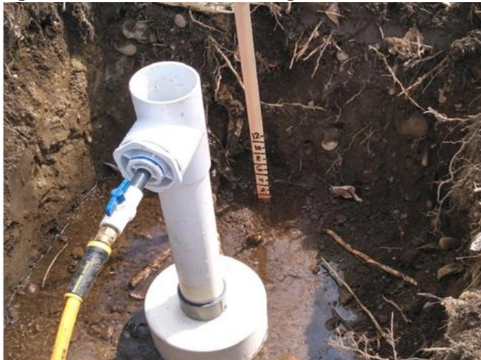
Figure 8: Infiltration Test in Progress PIT 3, Lot D
