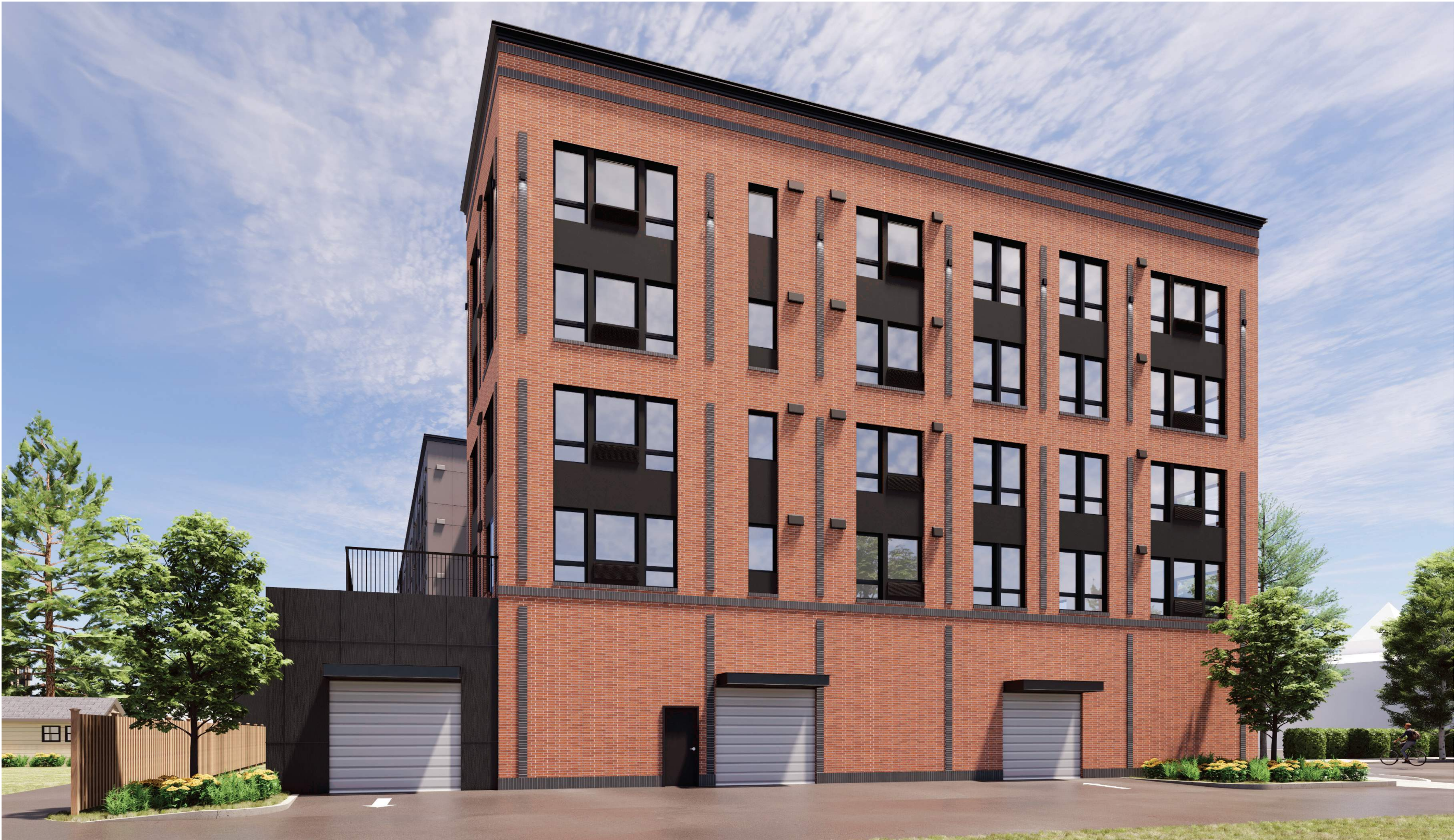
South Facade - Along alley
