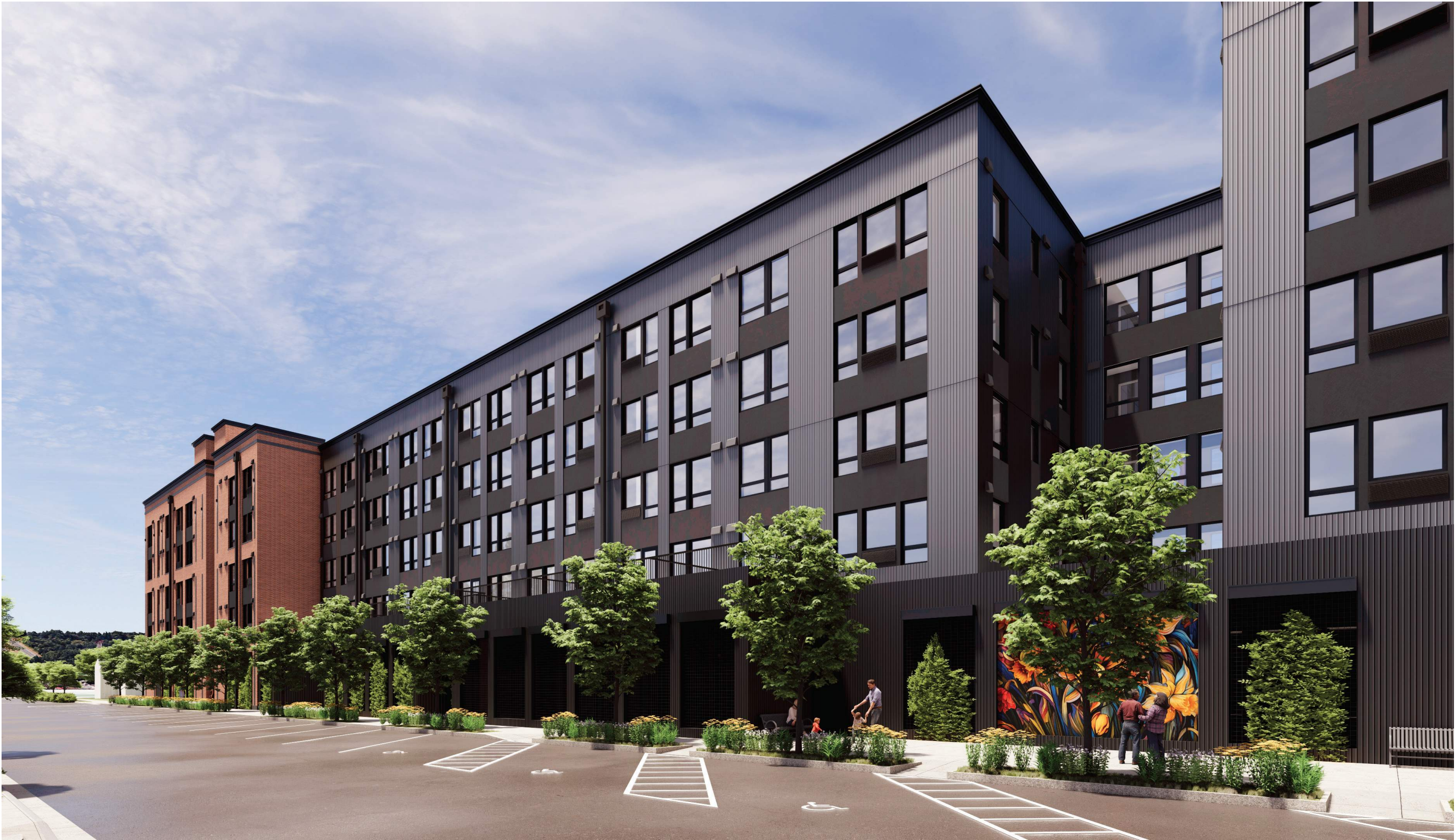
East Facade & Plaza - Along 3rd
