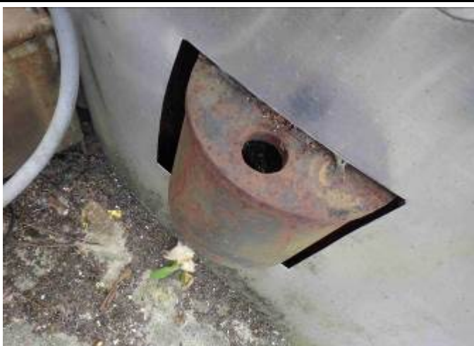
Missing Anchor Bolt
