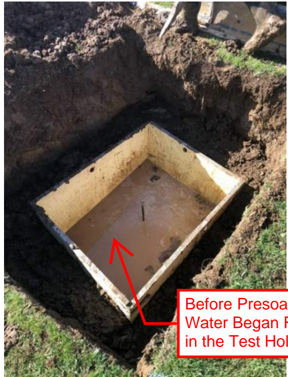
Groundwater Observed During Excavation
