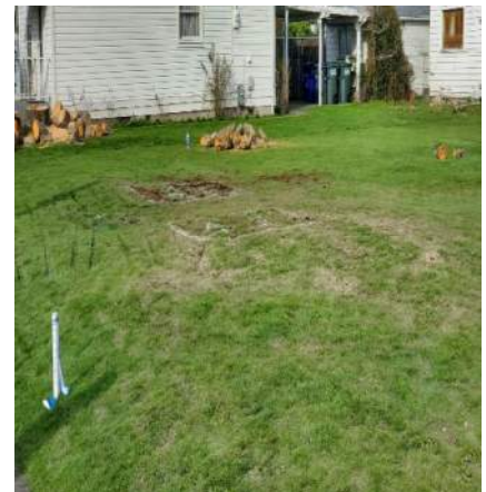
Backfill Test Hole
