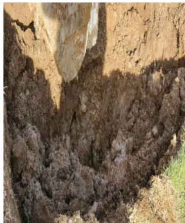
Over Excavation to observe if Groundwater is Mounding
