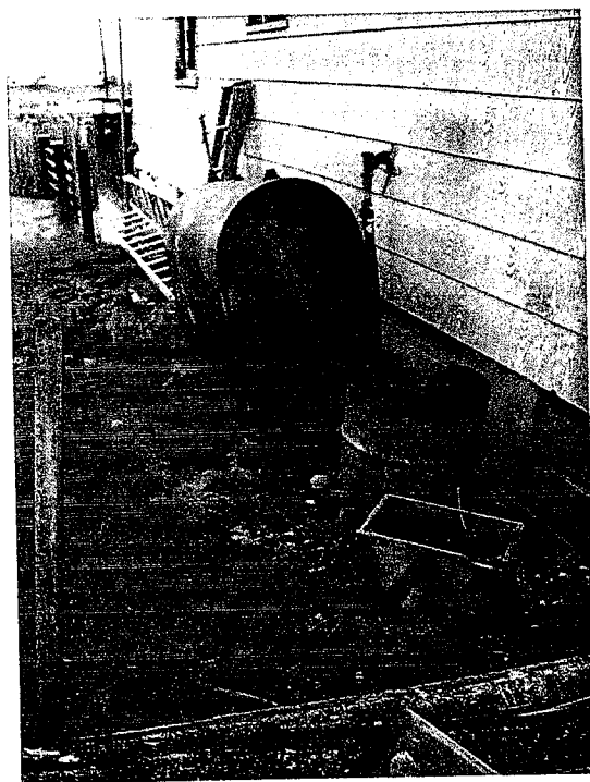
Photo 3: Heating oil tank observed adjacent to southern wall of northern house. Tank appeared to be in good condition.
