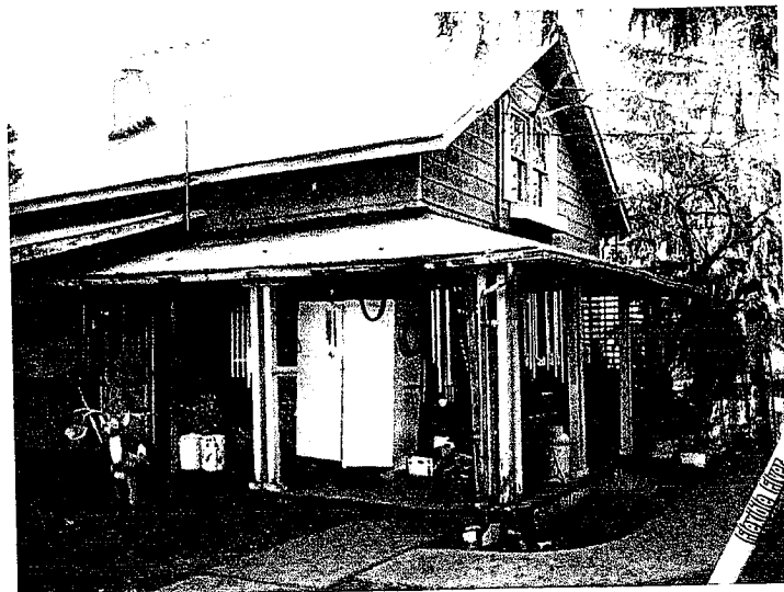
Photo 2: Northern house observed on subject site. Siding is asphaltic shingle material.
