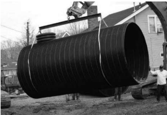
Lifting DuroMaxx into place with an excavator using nylon slings. When longer pieces are used, multiple nylon slings spaced 1/3 of the pipe apart should be used.
