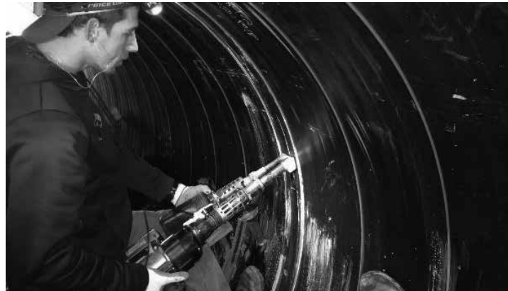
Internally welding pipe joints. The pipe needs to be backfilled prior to the joints being welded together. The pipe should be clean and dry. The gap between the two pipes should be limited to 1.5" maximum. The maximum pipe misalignment is 1/4". Pipe joints outside recommendations could result in higher joint welding costs.
