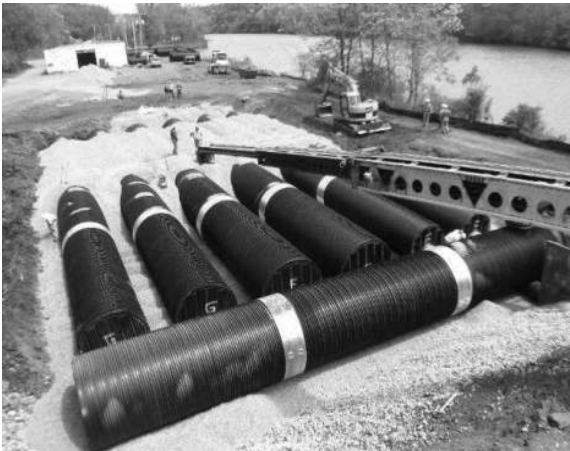
Placing backfill with a stone conveyor.
