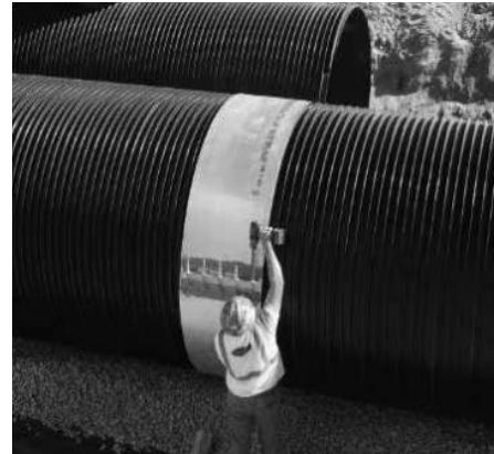
Tightening bolts on a flat band.
