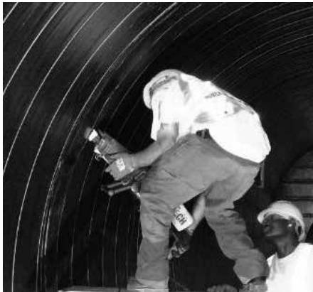
Internally welding pipe joints. The pipe needs to be backfilled prior to the joints being welded together. The pipe should be clean and dry. The gap between the two pipes should be limited to 1.5" maximum. The maximum pipe misalignment is 1/4". Pipe joints outside recommendations could result in higher joint welding costs.
