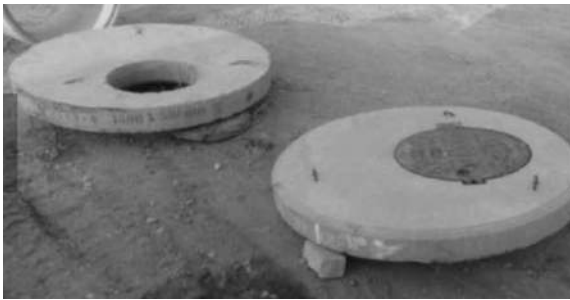
Precast option for manhole riser caps.
