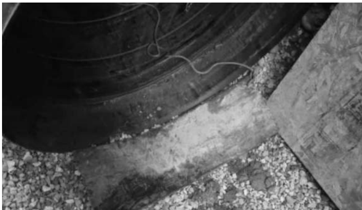
A best practice for bell and spigot joints is to lay a steel plate under the bell to help "home" the next pipe.
