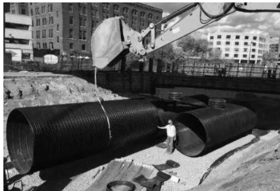
Lifting DuroMaxx into place with an excavator using nylon slings. When longer pieces are used, multiple nylon slings spaced 1/3 of the pipe apart should be used.
