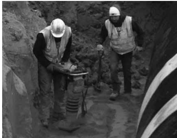
Compaction with vibratory equipment.
