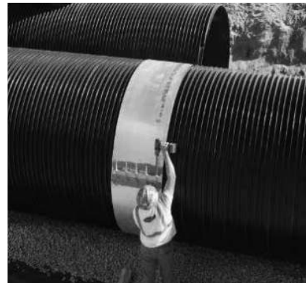
Tightening bolts on a flat band.
