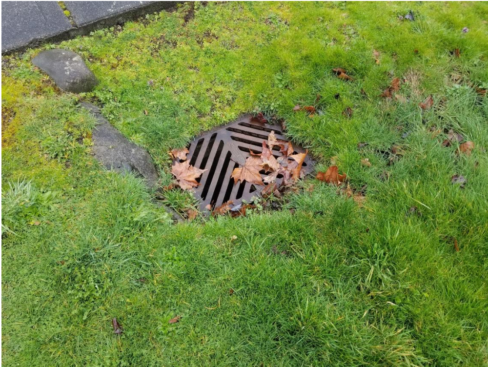
Photo 20—Catch basin inlet near 14 th Street SW.
