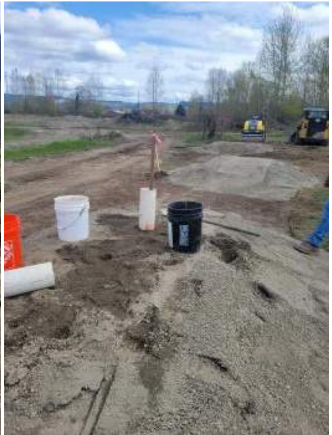
UPLOADED: 04/04/2022 14:07:45 Miles Pit Run - Gravel Borrow
