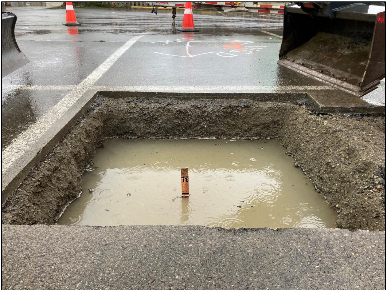
Figure 2: Small-Scale PIT Excavation
