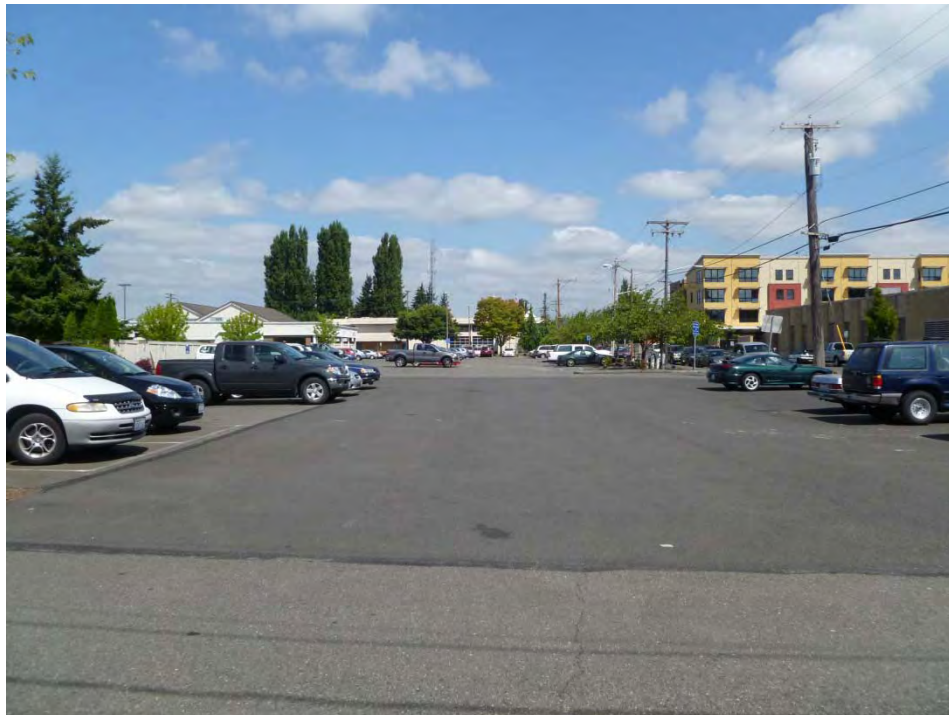
LOOKING NORTH ACROSS EAST SIDE OF PROPERTY PATCHED ASPHALT IN FOREGROUND IS FORMER BUILDING LOCATION
