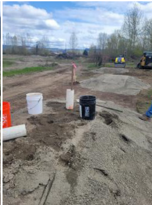
UPLOADED: 04/04/2022 14:07:45 Miles Pit Run - Gravel Borrow
