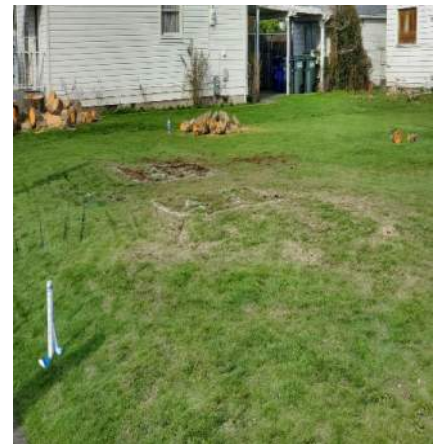
Backfill Test Hole
