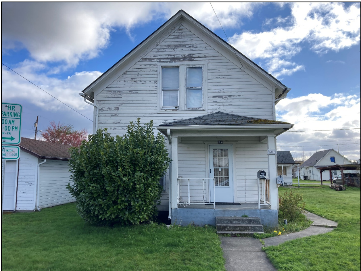
Figure 5. Front (east) view of building at 607 3rd St. SW.
