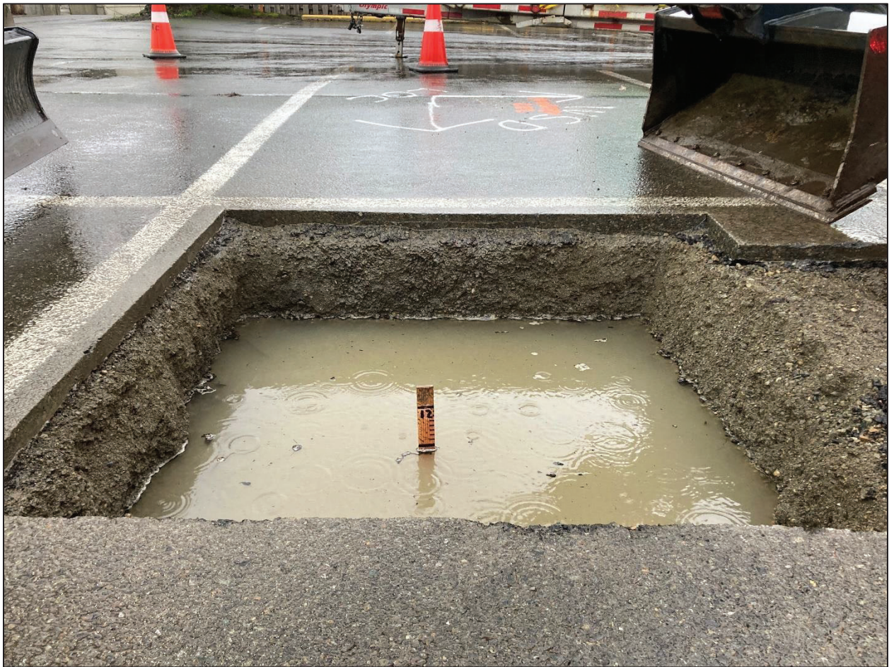
Figure 2: Small-Scale PIT Excavation
