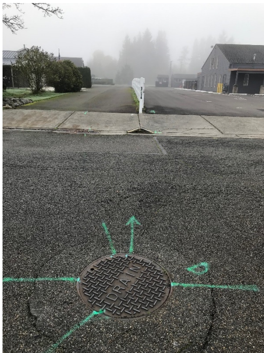
The above left photo shows the existing storm manhole located on 9th Ave SW approximately 250 feet east of the intersection. Once runoff reaches this manhole, it begins to flow south for approximately 500 feet through an existing public storm easement running along the Puyallup Community Baptist Church property. Runoff then flows westward for approximately 80 feet and enters the existing pump station shown in the above right photo.
