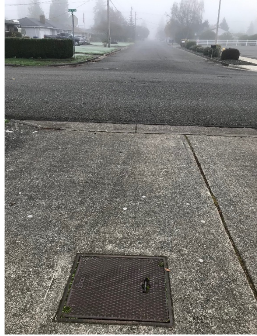
The above photos show the downstream catch basin at the intersection of 14th St SW and 9th Ave SW. Once runoff reaches this catch basin, it begins to flow east along 9th Ave SW for approximately 250 feet. The above right picture shows the catch basin looking east towards 9th Ave SW.
