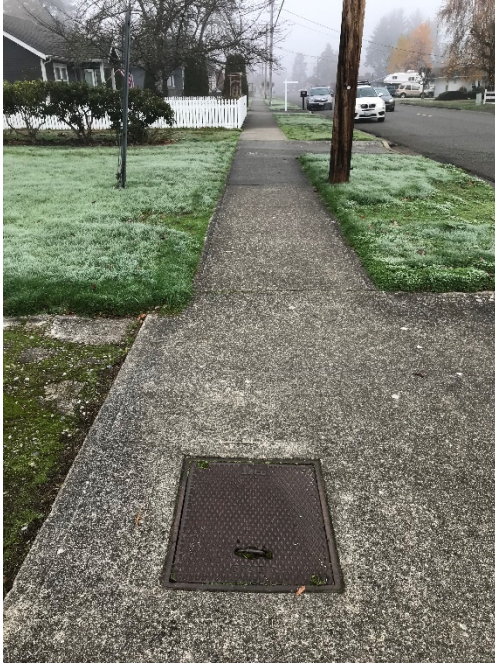
The above photos show the downstream catch basin at the intersection of 14th St SW and 9th Ave SW. Once runoff reaches this catch basin, it begins to flow east along 9th Ave SW for approximately 250 feet. The above right picture shows the catch basin looking east towards 9th Ave SW.
