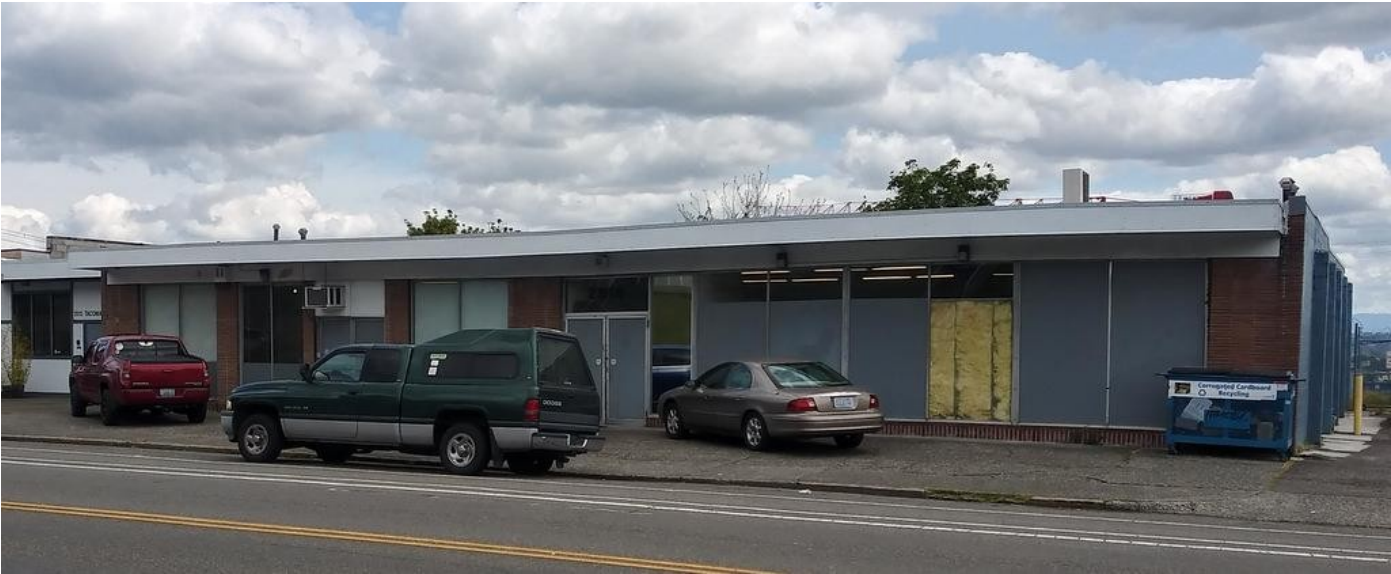
Fig. 1 – Located along Tacoma Avenue, Tacoma, WA
