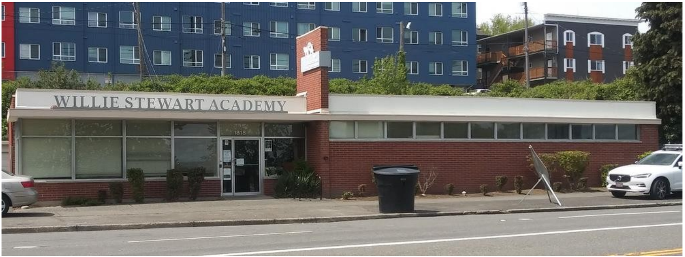
Fig. 3 – Located along Tacoma Avenue, Tacoma, WA
