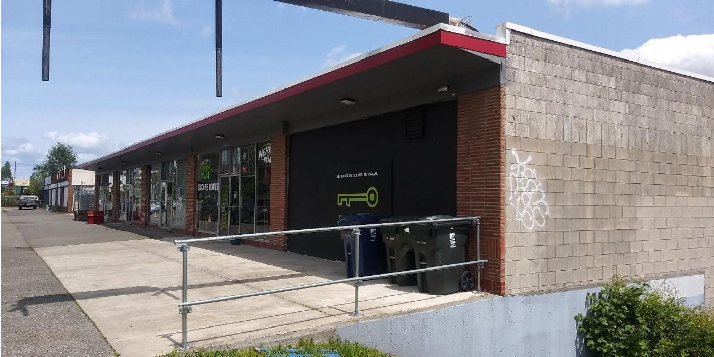
Fig. 2 – Located along Tacoma Avenue, Tacoma, WA
